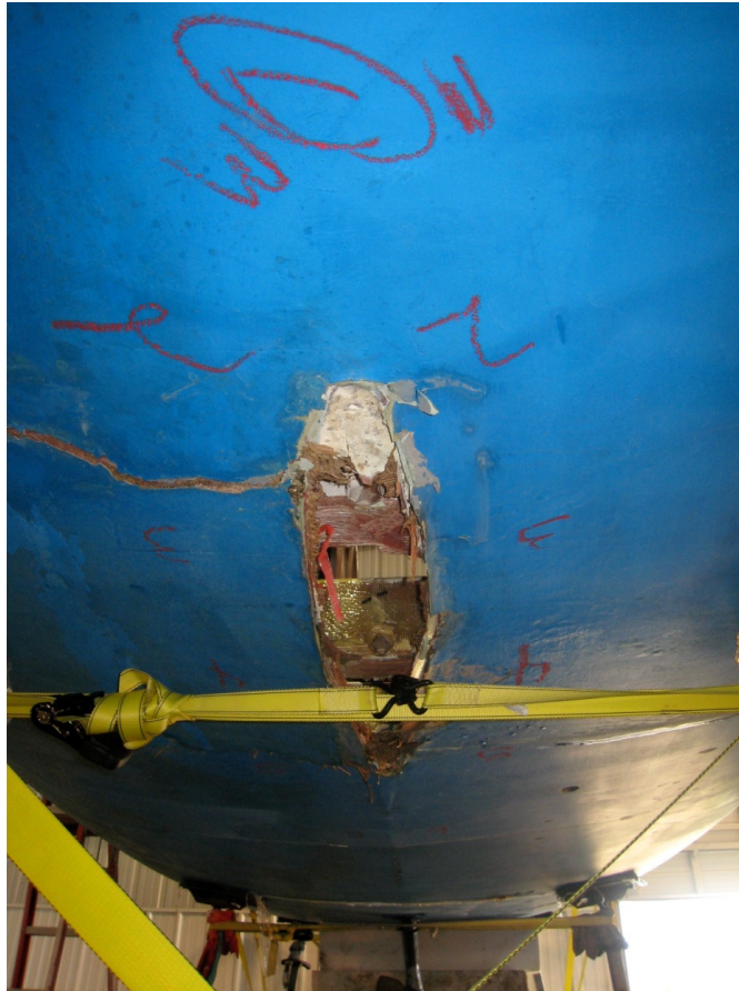
View looking up at where the keel should be
