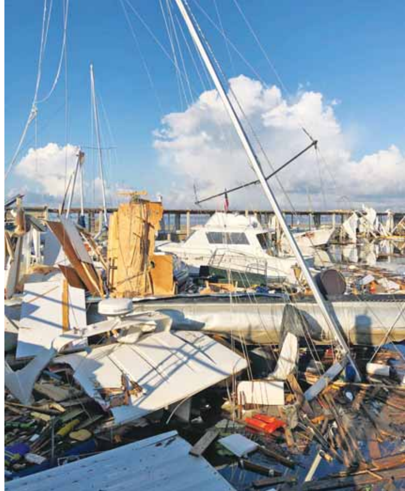
The Panama City Docks were unrecognizable following the beating by Hurricane Michael. Pieces and parts of boats were tossed everywhere.
