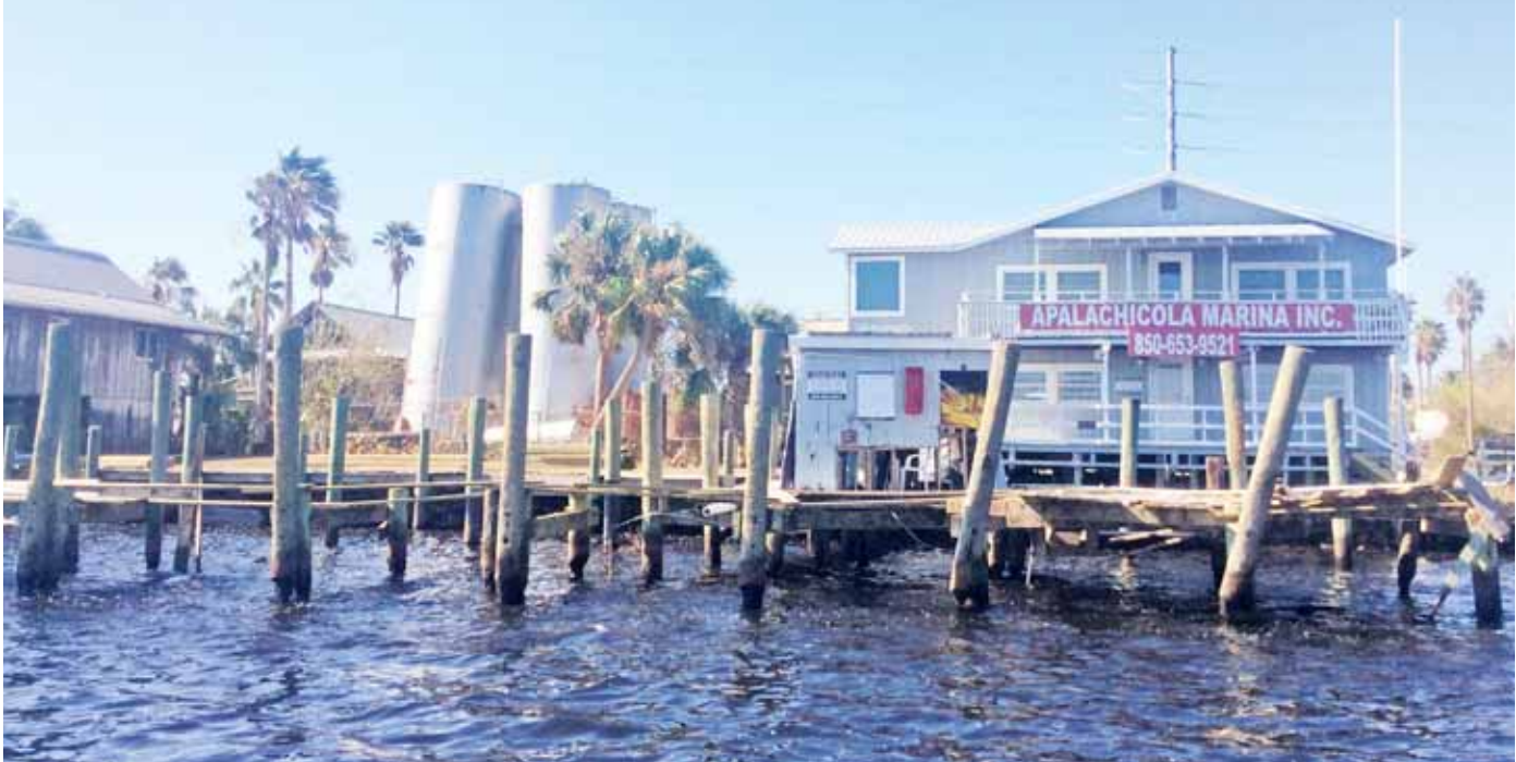
Apalachicola Marina fuel dock was mostly destroyed. The fuel tank in the background is leaning.
