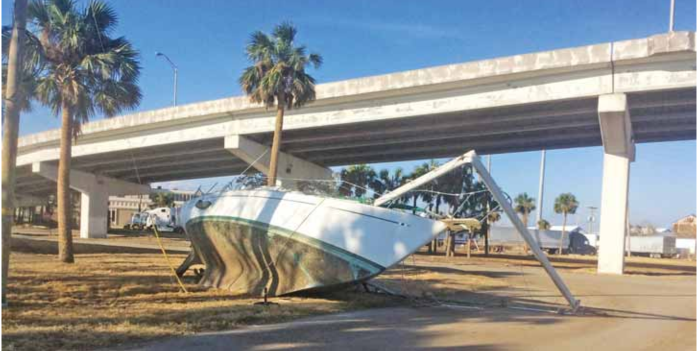
A sailboat, about 35 feet long, moved from its dock in Ten-Foot-Hole marina across the street, about 200 ft. from its dock. The piers and boardwalks at Ten-Foot-Hole were damaged and will require repair.
