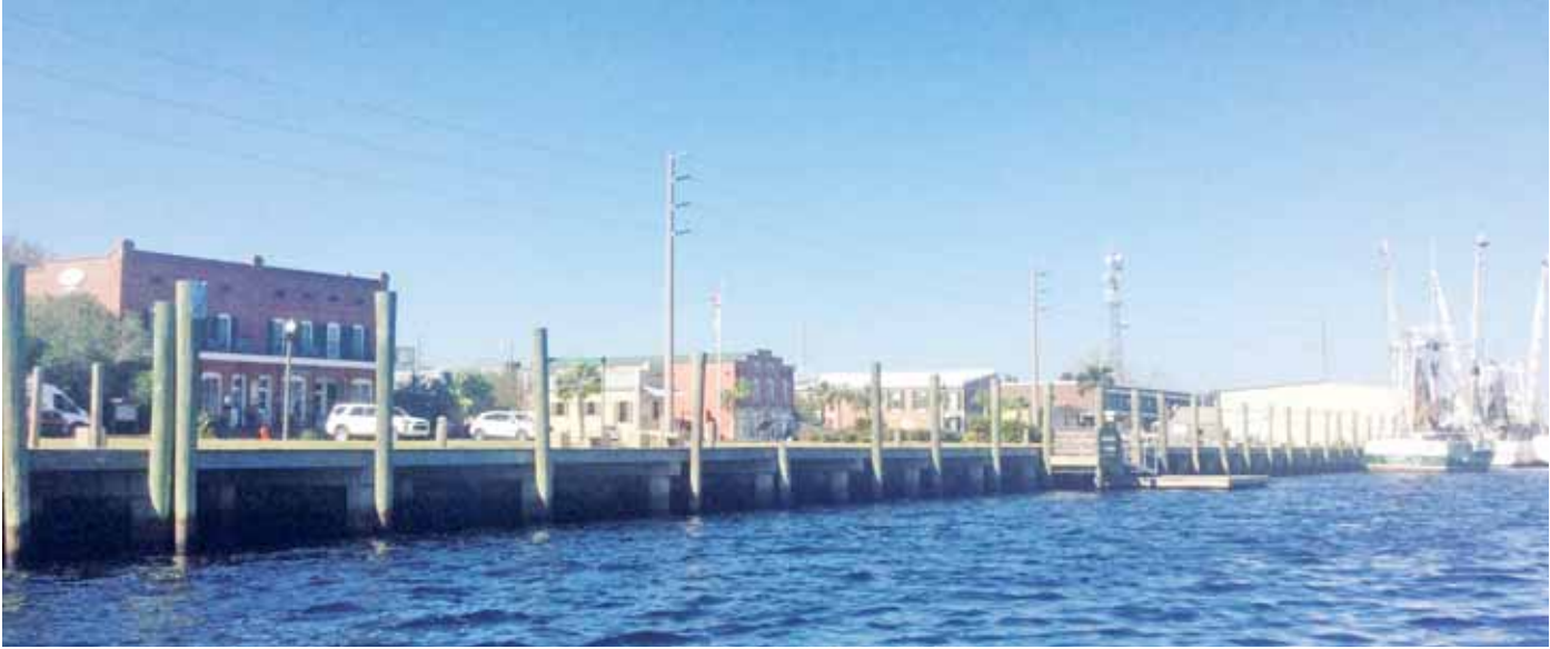
Although large mounds of debris were washed ashore and mud covered the downtown streets, Apalachicola Riverfront Park suffered almost no damage.
