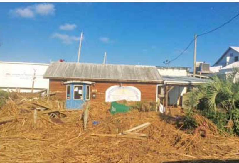
Seagrass and debris deposited on Water Street (which runs along the waterfront) by storm surge, but the small building behind still stands.
